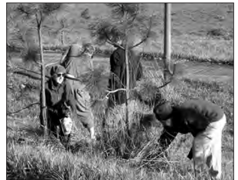
Maintenance work at Westmoreland Park on January 23, 2010.
